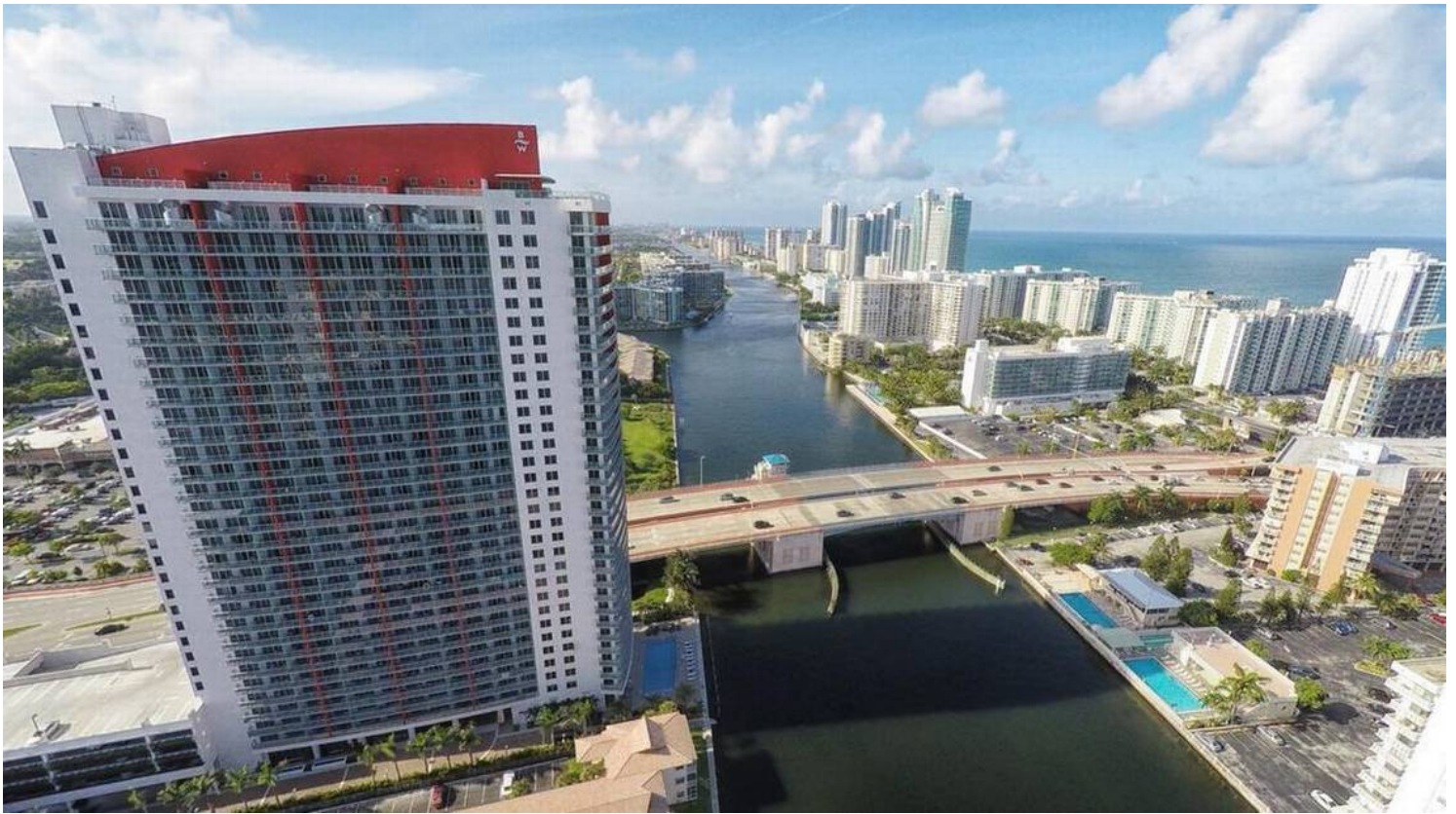
High-rise condos line the shores of Hallandale Beach in southern Broward County. Miami Herald file photo
